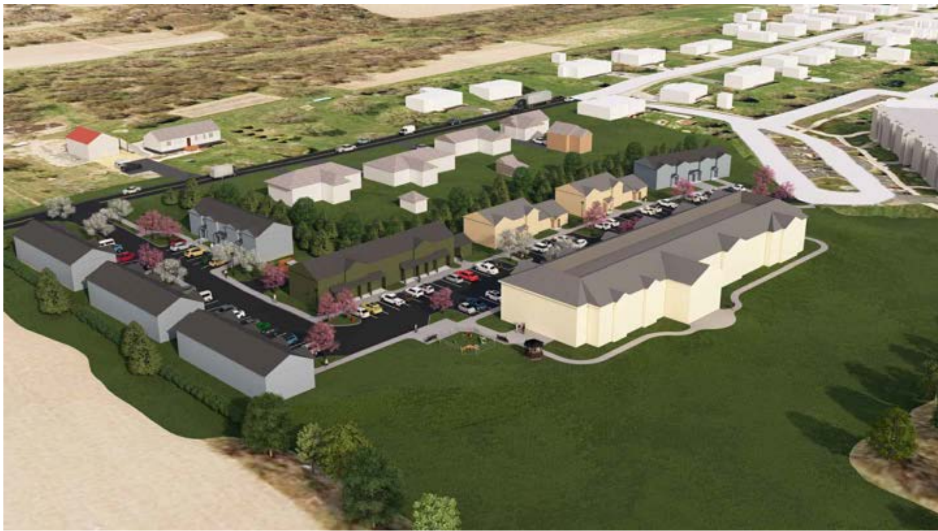
3: LOOKING SOUTHWEST AT PERU ROAD & PROPOSED DEVELOPMENT
